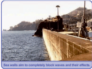
Sea walls aim to completely block waves and their effects.
